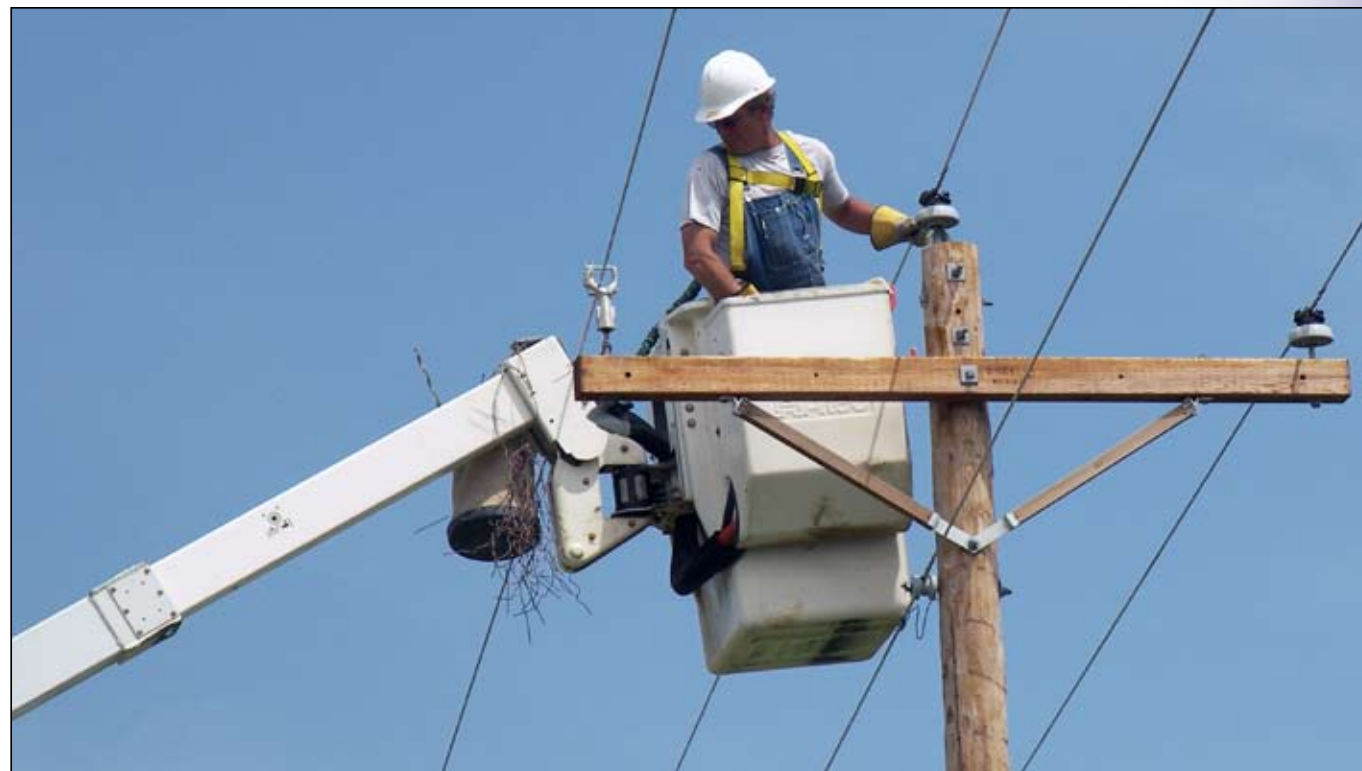
Above: Lyon-Coffey Journeuman Lineman Steve Rohde installs an conductor on the line. Right: Bucket trucks line the highway to make necessary repairs at Virgil Metering Point.
