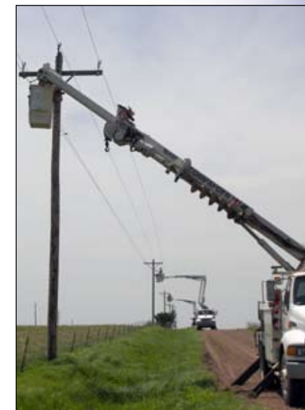
Above: Lyon-Coffey Journeuman Lineman Steve Rohde installs an conductor on the line. Right: Bucket trucks line the highway to make necessary repairs at Virgil Metering Point.
