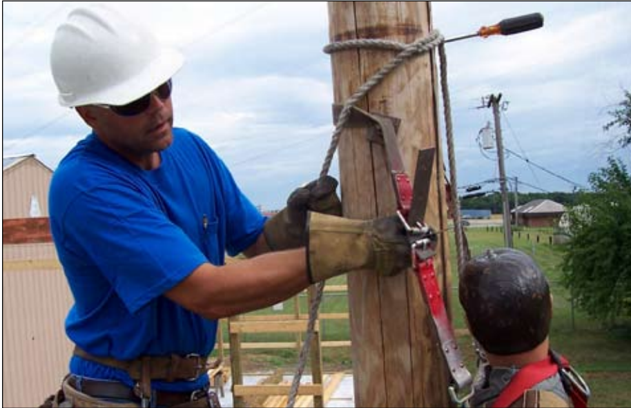
Mark Doebele tightens the safety harness around the training dummy during the pole-top rescue exercise.
